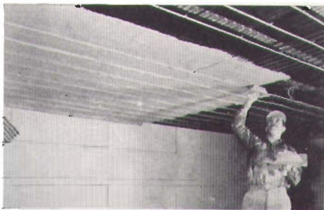
Applying the first or scratch coat of Gypsum plaster to ceiling. Other coats will follow to give final cover of \frac{1}{4} " over copper tube.
