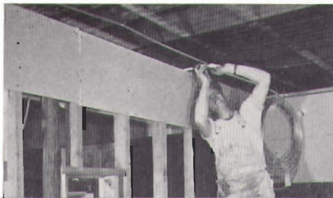
Locating the position of the first tube in the ceiling panel coil. Notice the coil of copper tube temporarily hung from the mesh with a U-hook while the measurement is being taken.
