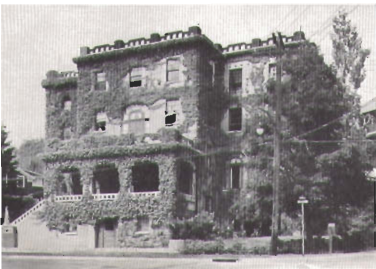
In 1910 the Cornell Cosmopolitan Club was one of the first Radiant Heating installations in this country.
