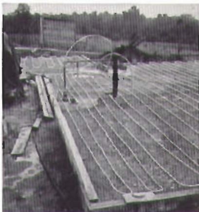
Approximately 1,200 ft. of 3/8" Type L Copper Tube was built into panel coils for this house.
